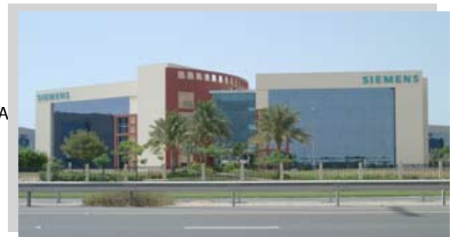
SIEMENS BUILDING-INTERNET CITY - Dubai
