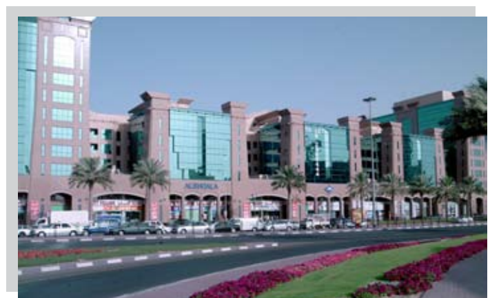
Project : AL SHOLA COMPLEX, Dubai
