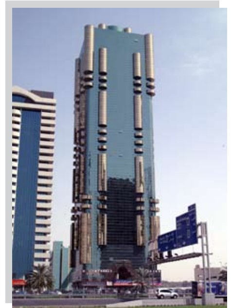
Project : AHMED AL ATTAR TOWER, Dubai Client : MR. AHMED AL ATTAR Consultant : M/S. AL THURATH CONSULTANT
